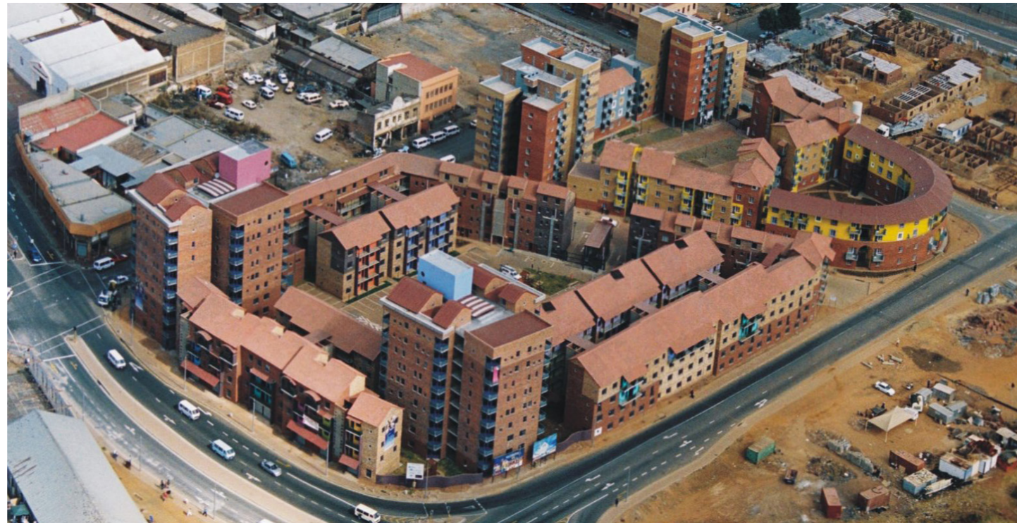
Figure 7.4: Brickfields and Legae social housing project, Johannesburg ( http://savagedodd.co.za/wp-content/uploads/2017/05/aerial-view-2048x758.jpg )
