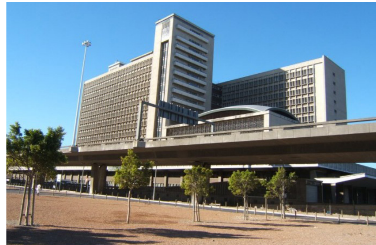
Figure 7.8: Customs House building ( http://saarcimag.weebly.com/uploads/1/3/4/3/1343219/7146115_orig.jpg )
