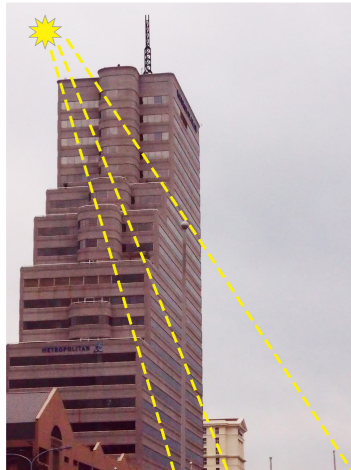
Figure 5.22: Height setbacks of the Metropolitan building in Cape Town allow more sunlight to reach the street (Author, 2017)
