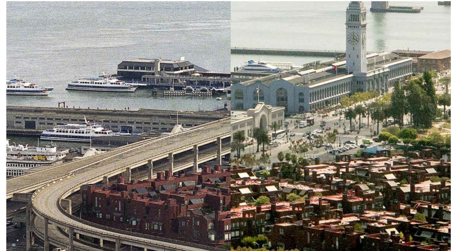
Figure 7.2: San Francisco Embarcadero before and after the removal of the elevated freeways. ( http://media.bizj.us/view/img/4024951/embarcaderooverviewslidertease*1200xx1761-991-0-163.jpg )
