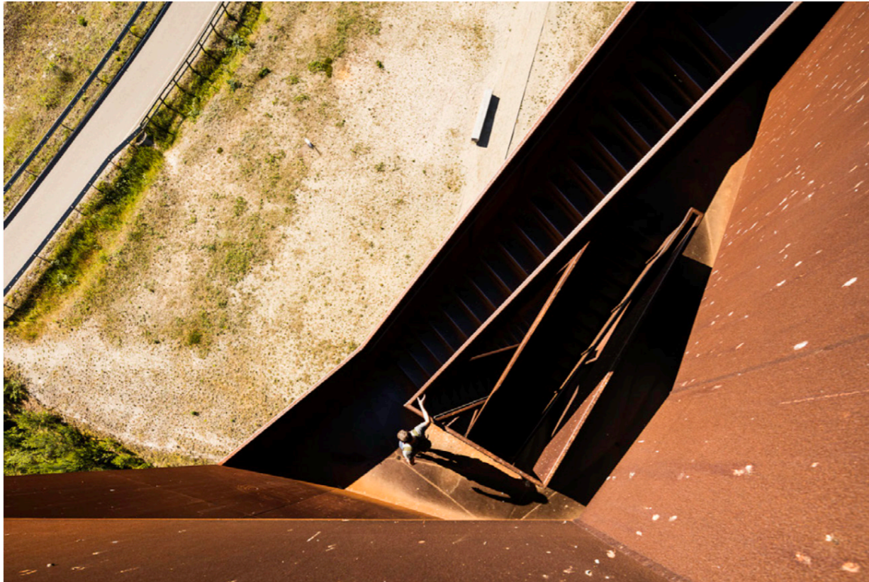
Framing stringers imbuing safety from height (Figure.37) (Stefan Giers) (Börner, 2008)
