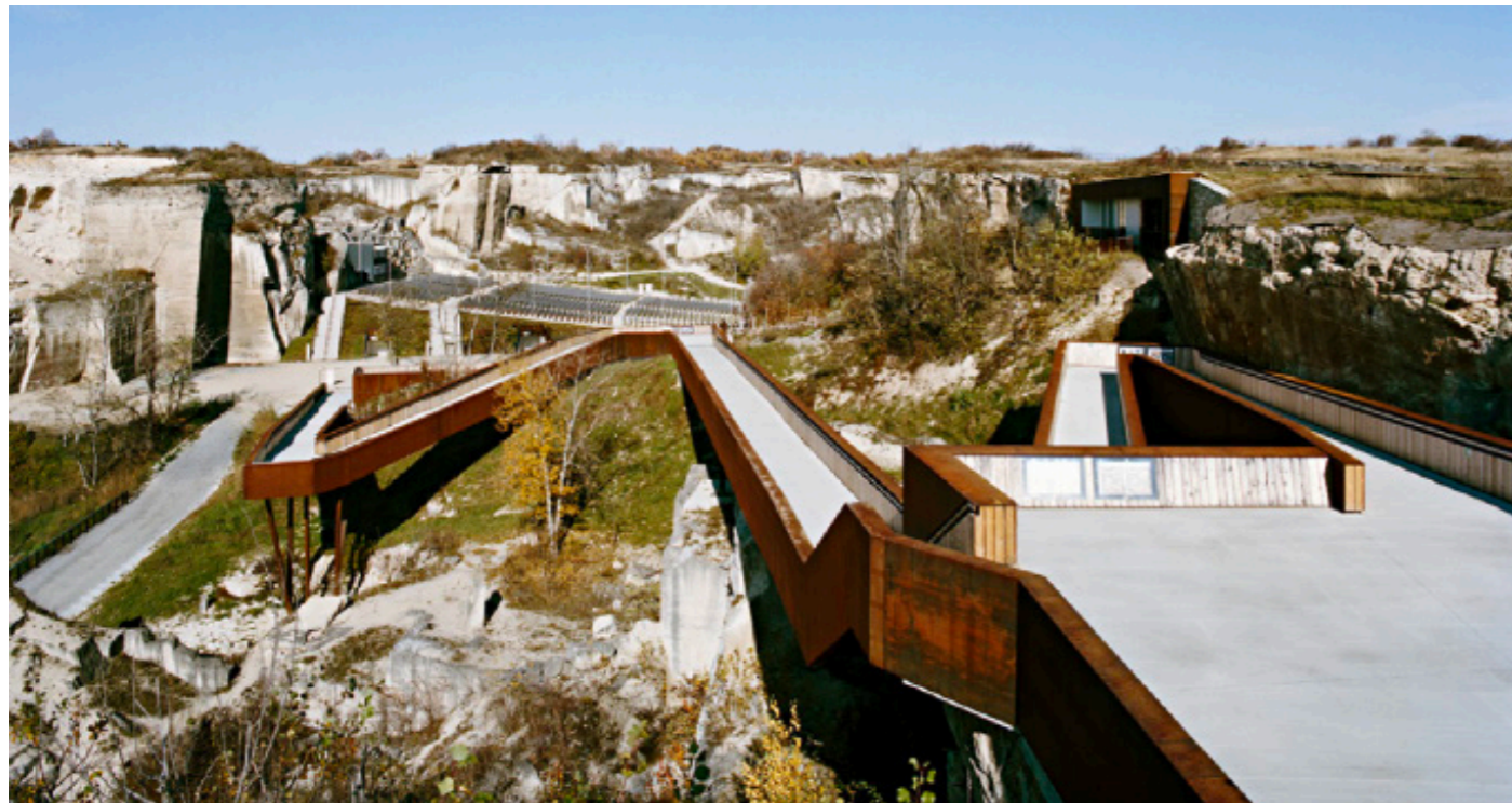
Elevated walkway (Figure. 40) (Hertha Hernaus) (Seip, et al., 2013)
