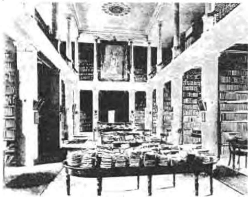
135. The National Library of South Africa, view of the interior of the reading room, (Picton-Seymour, D, Victorian Buildings in South Africa, including Edwardian & Transvaal Republican Styles 1850 -1910 , A.A. Balkema, Cape Town, Rotterdam, 1977, p.40)
