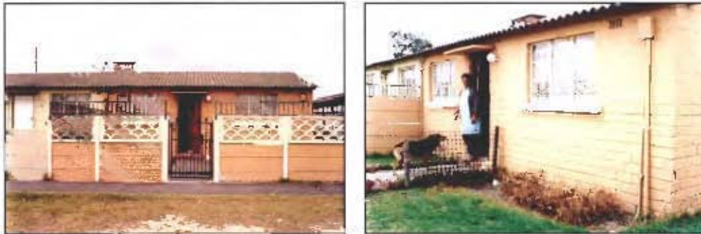
Figure 3-8: A council house in Mannenberg, Cape Town that was used as a reference for the virtual house.
