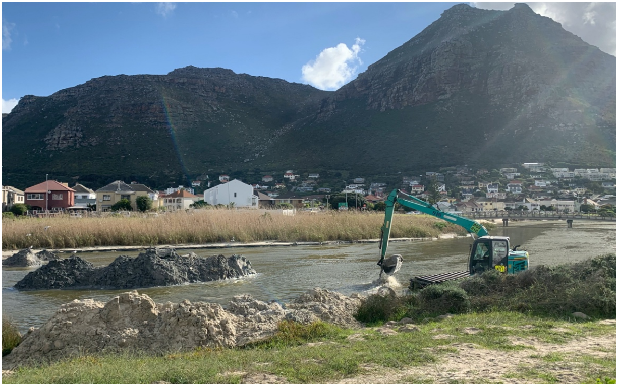
Figure 4: Dredging in Zandvlei Estuary, captured on 27 August 2021 by Carla de Cerff
