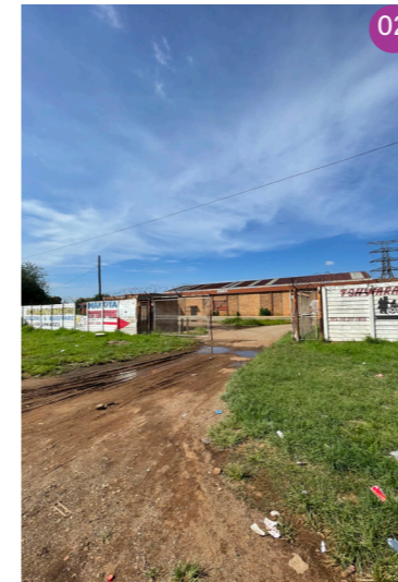
Figure 05: Signs of urban decay along Ikageng Gateway corridor (source: author's own, 2024).
