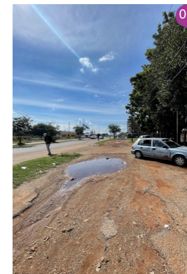
Figure 06: Signs of urban decay along Ikageng Gateway corridor (source: author's own, 2024).
