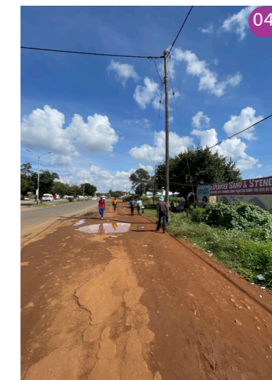
Figure 07: Signs of urban decay along Ikageng Gateway corridor (source: author's own, 2024).
