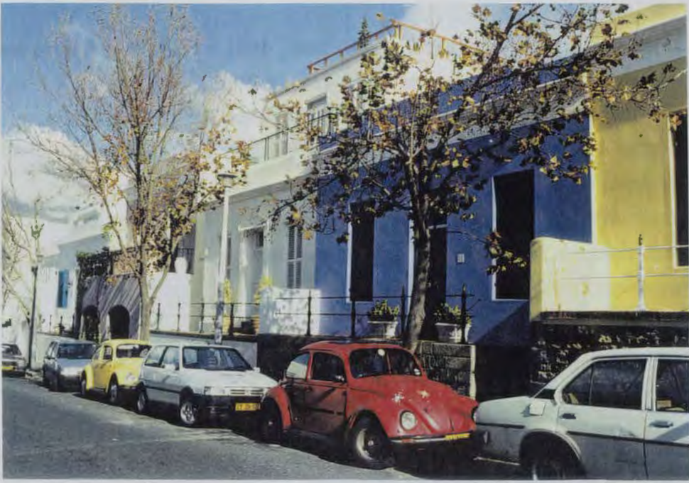
Figure 4.8: Picture 1 - The De Waterkant area today (This photograph (of a present-day De Waterkant street scene) depicts a gentrified 'upmarket' inner city area. The embellishment and ornamentation of these vernacular Cape 'Malay' cottages clearly reflect the (post)modern tastes of their new residents).
