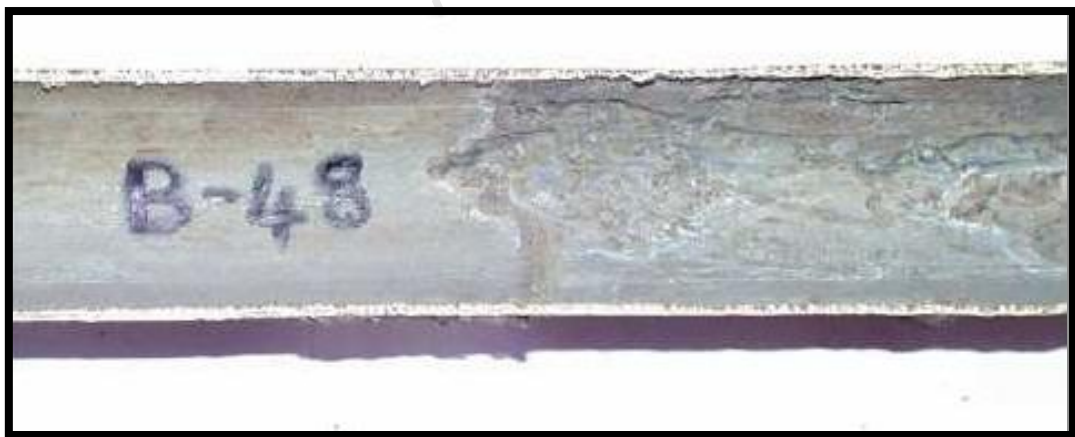
Figure 2.10: Internal erosion over long length [17].
