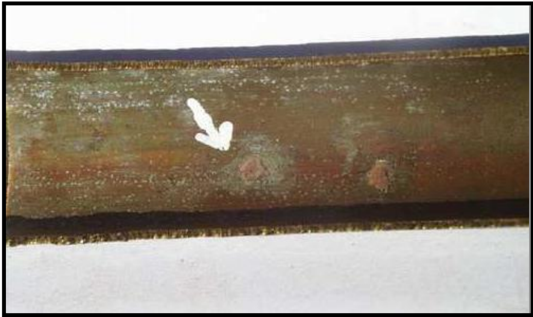
Figure 2.6: Internal pits filled with corrosive product [18].
