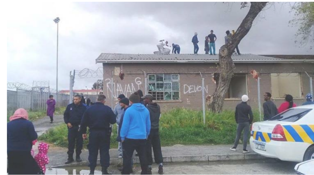
Figure 57: Before: The Old Rent Office, located along Manenberg Avenue, was remaining idle for far too long.
