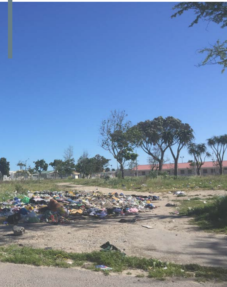
Figure 50: Marico Park, upgrade and tree planting partially completed at the swimming pool. Contractor walked off site - park slowly being vandalised and becoming a space to dump rubbish and waste. (author's own)
