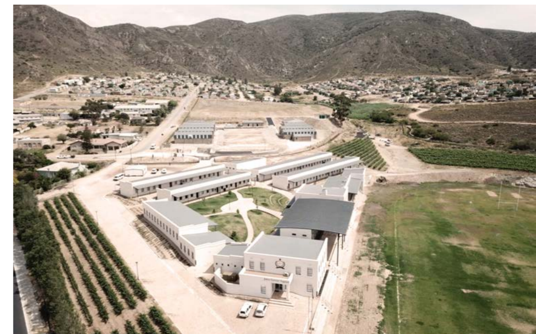
Figure 169: Jakes Gerwel Technical School, Bonnievale, Western Cape. The design incorporates a stimulating educational environment, which encourages access to programmes and shared facilities. The project was born out of the community to address the needs of students for a technical training resource in the under-served farming community.
