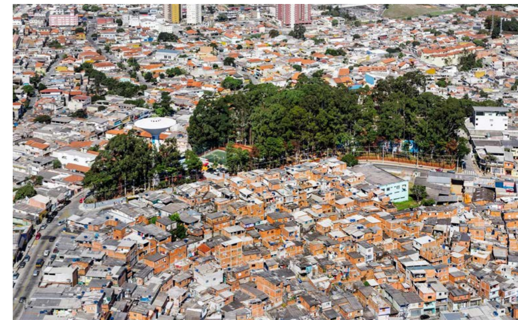
Figure 126: Linear park spaces occupy small strips of land between the dense slums in Sao Paulo. These networks adapt any seemingly unoccupied parcels and create around and with the space. Shown in this image is a linear park built around water tanks and reservoirs, ensuring all available space is optimised and occupied.
