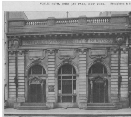
FRONT FACADE (Image: Renner, 2008, p.509)
