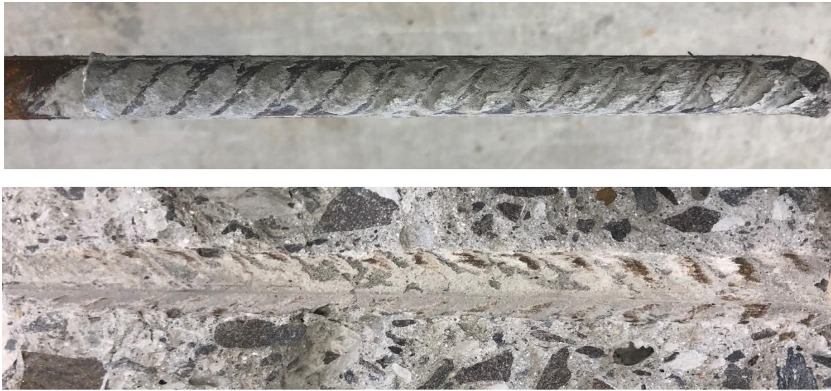
Figure 33: Coating remains and concrete-steel interface after failure
