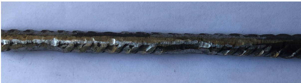
Figure 20: 10% cleaned corroded steel
