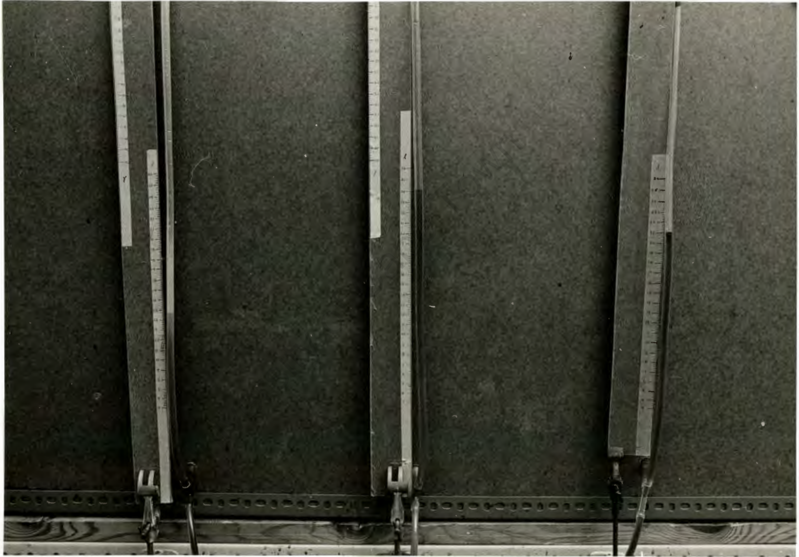
Fig. 3.11 Sight Tubes Indicating Liquid Level in the Feed Tanks.
