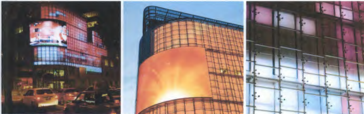
Fig 40: The A.AMP facade of a Singapore office building
