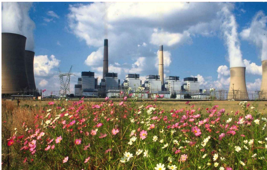
Figure 1: Exterior view of Kriel Power Station [10]
