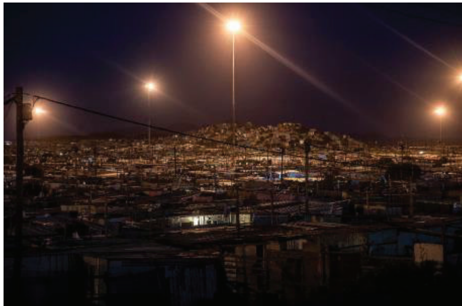
Figure 4.6: Image showing poor illumination between shacks due to high-mast public lighting in informal areas in Khayelitsha. Data Source: Wang, 2022
