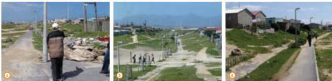
Figure 96 Poor maintenance of public lighting results in inadequate lighting levels at night time
