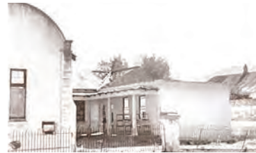
Biscombe, H. (2006d). Die Vlakte demolished [Photograph]. Stellenbosch.
