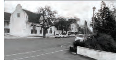
Site visit image taken in Plein Street
