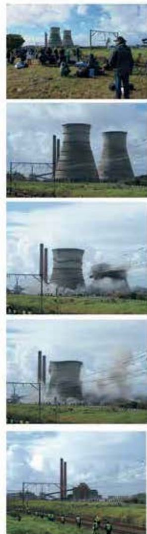
DEMOLISHING OF COOLING TOWERS
