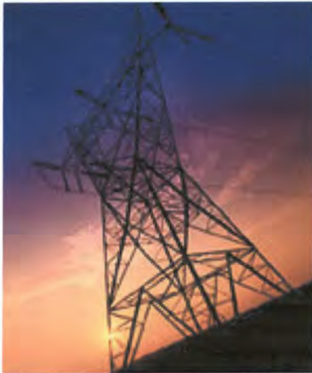
Electricity pylon (Photograph: Oliver Wood)
