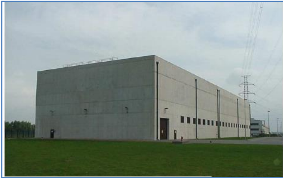
Figure 4-12: Cask storage building at Doel dry storage facility [122]
