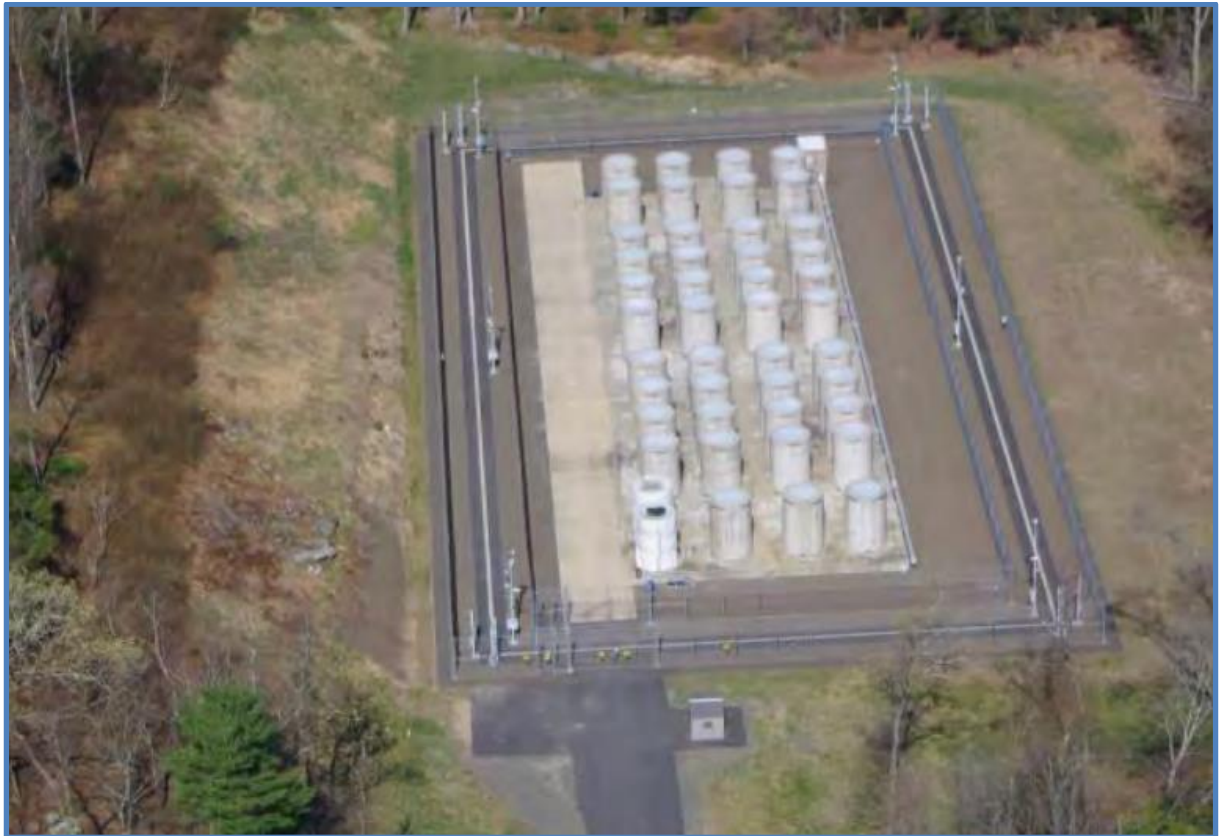
Figure 4-2: Aerial view of the Connecticut Yankee ISFSI at Connecticut Yankee adapted from [104]
