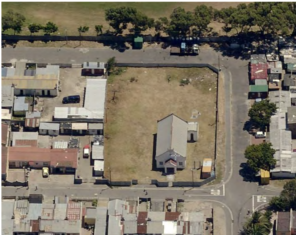
Figure 19: Oblique aerial view of AME Church in its context (CCT – ISIS)
