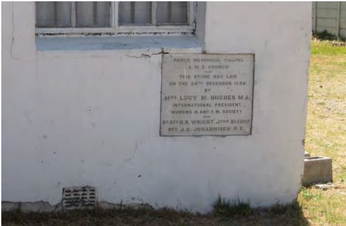
Figure 23: Foundation stone on front corner dated 24 December 1938
