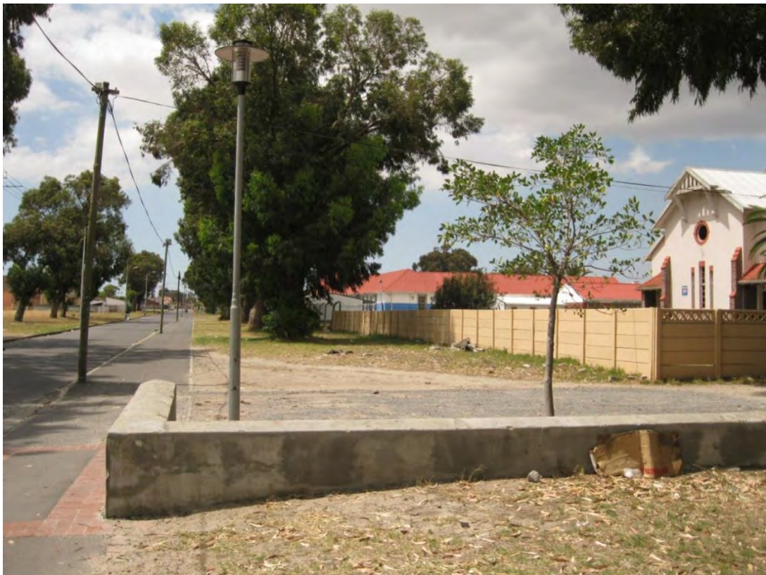
Figure 15: Position of church in relation to street (Lerotholi Avenue)
