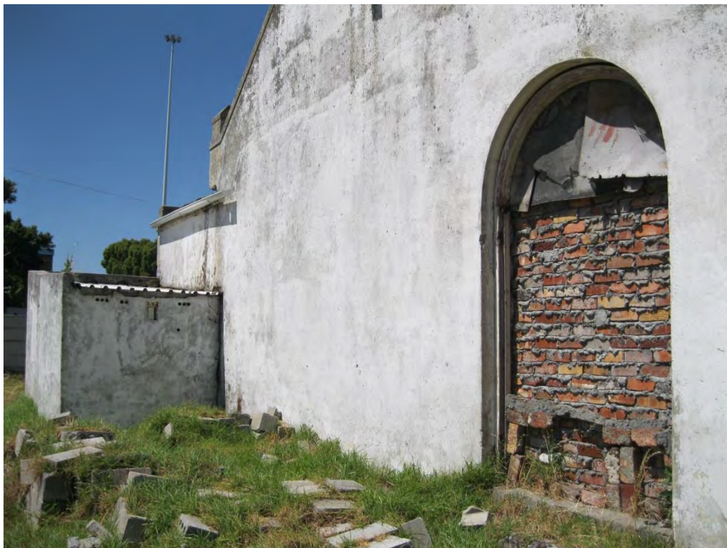
Figure 22: Back of the church showing former external door bricked in
