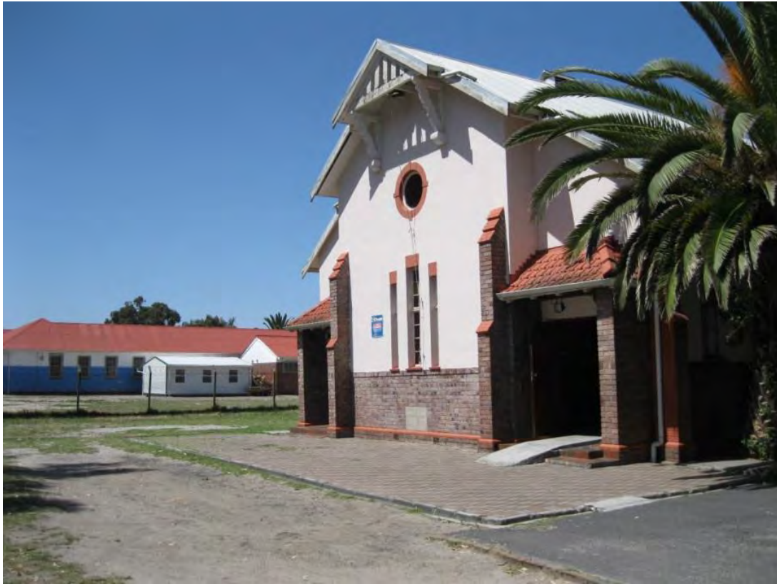
Figure 14: Front facade of Wesleyan Church
