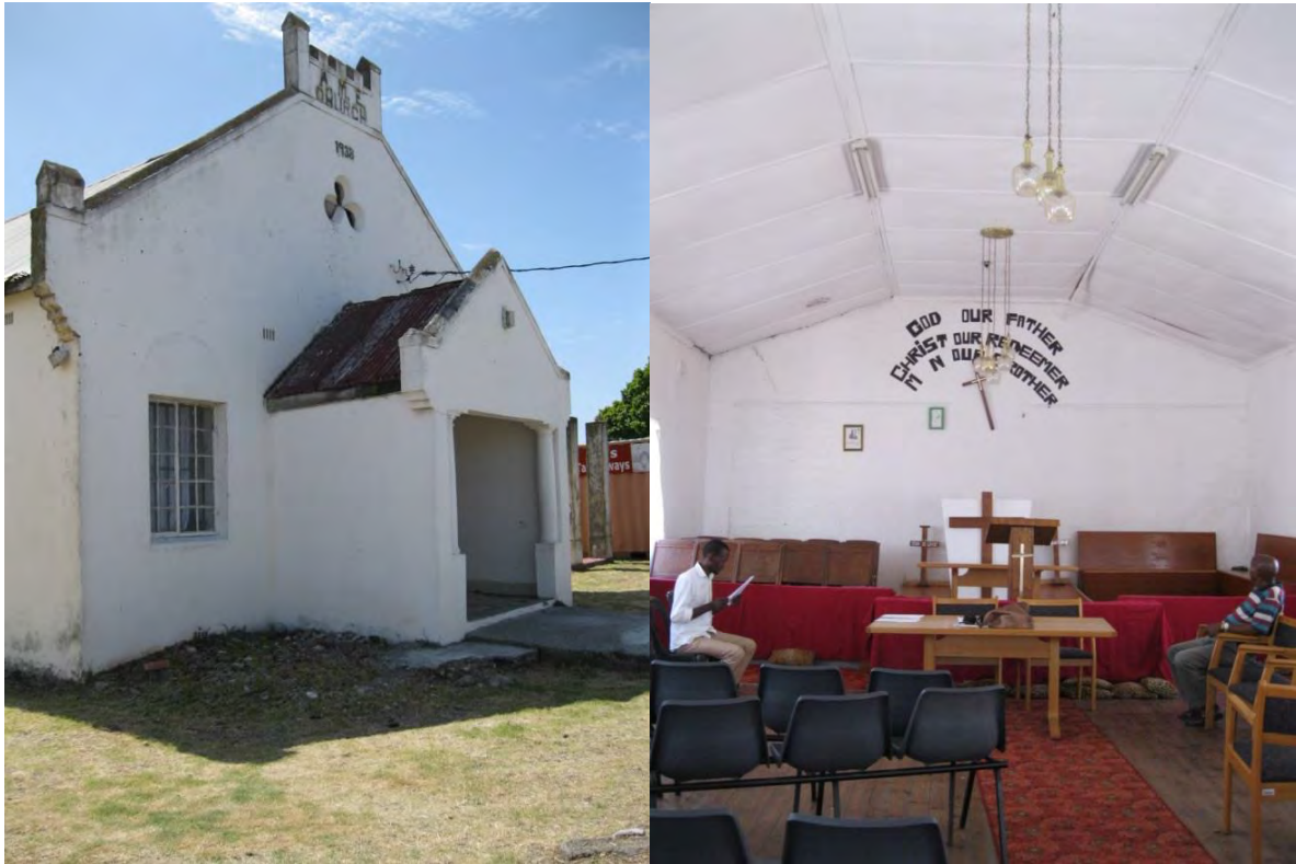
Figure 20: The front entrance of the AME Church (left)
