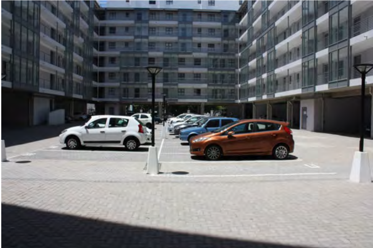
Figure 3-8: Image of RPPS. The PPS covers the parking bays only, while the remainder of the pavement is impervious
