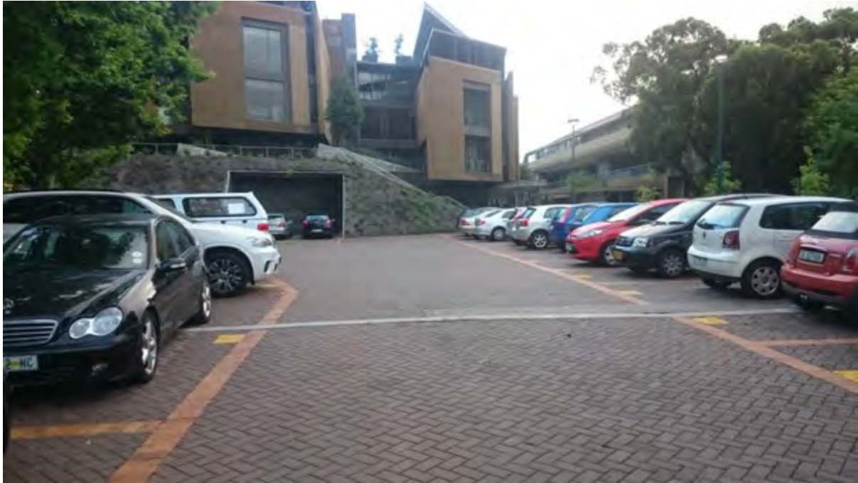
Figure 3-5: Picture of the NEB PPS. Note the ground beam separating PPS sections in the middle of the picture
