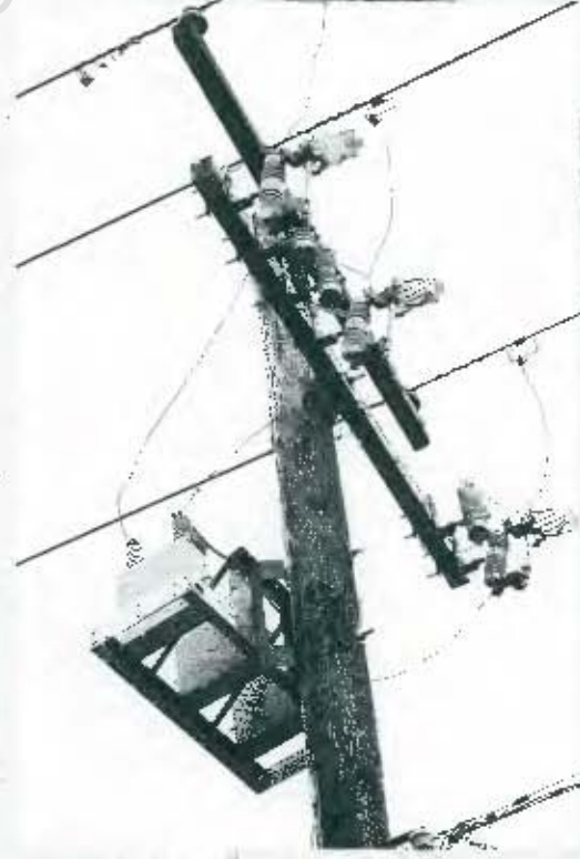
ABB cutouts protect capacitor banks against overcurrents, visibly indicate when equipment is energized, and interrupt capacitive currents.
