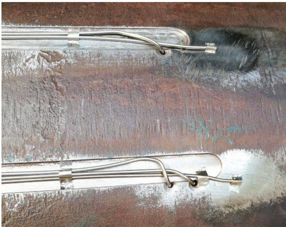
Figure 99. Thermocouple installation - Position A and B
