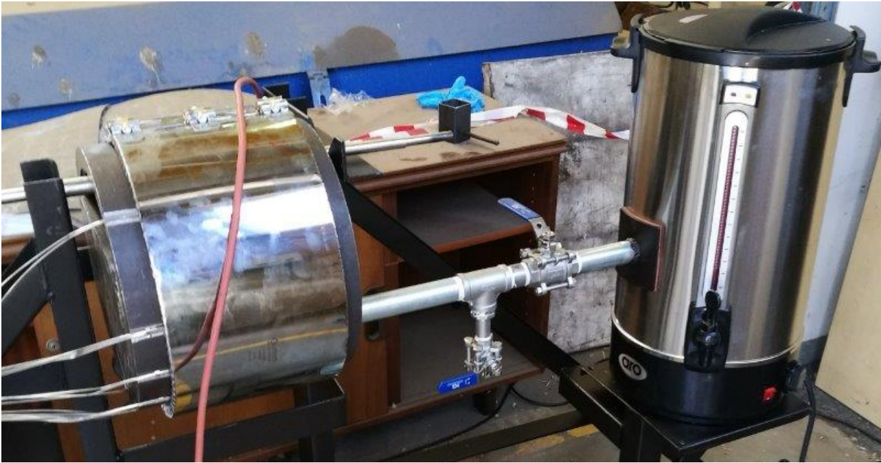
Figure 97. Ceramic band heating element fitted over the steam pipe (left) and water supply from Urn (right)
