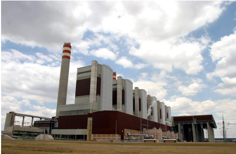
Figure 1. Power Station A
