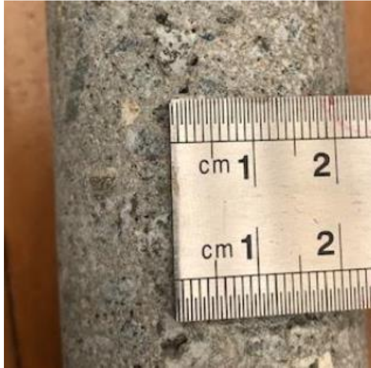
Figure 4.2: Image showing visible entrapped air (compaction void) on a core sample used in density measurements
