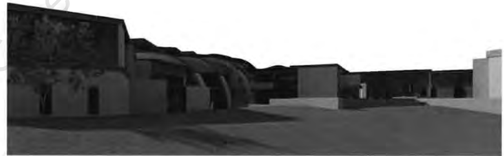
Below: North facade showing the structural ribs and buttresses
