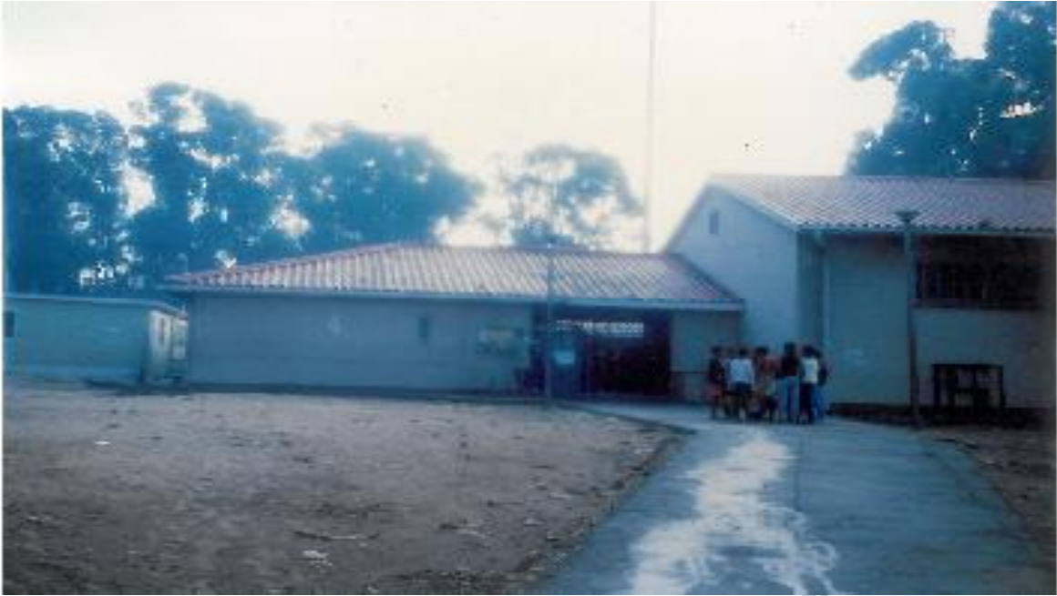
Plate 2.4 Front view of Zolani Center
