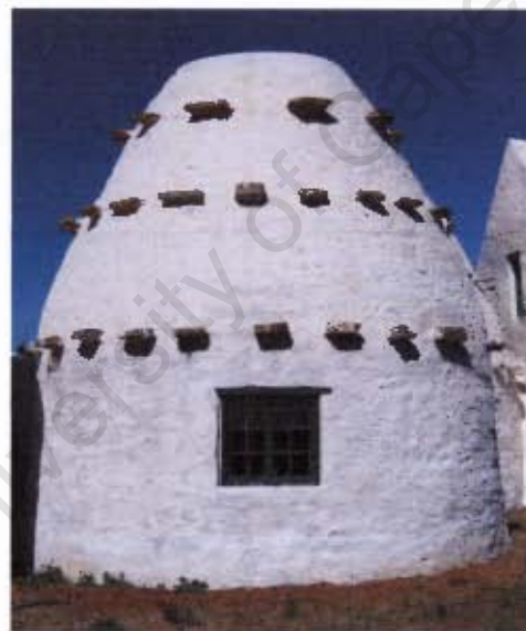
Figure 4.35 Stuurmansfontein I. The rows of projecting stones are too far apart to allow the builder or repairer to easily step up from one level to the next.
