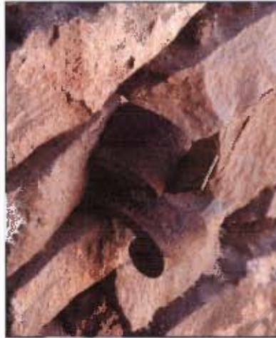
Figure 4.53 Omkeerkolk. Metal in the doorway used to attach a form of door.
