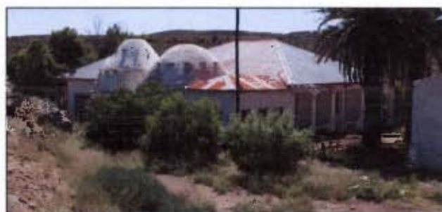
Figure 6.45 Konka. The corbelled buildings have been enveloped by the 1950s building.
