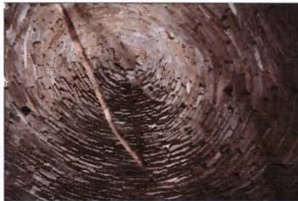
Figure 4.23 Brakvlei Perfectly built roof with a small root hole.
