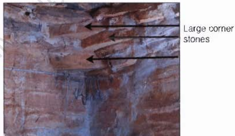
Figure 4.14 Brownslaagte. Large corner stones enable the square base to carry the round roof.
