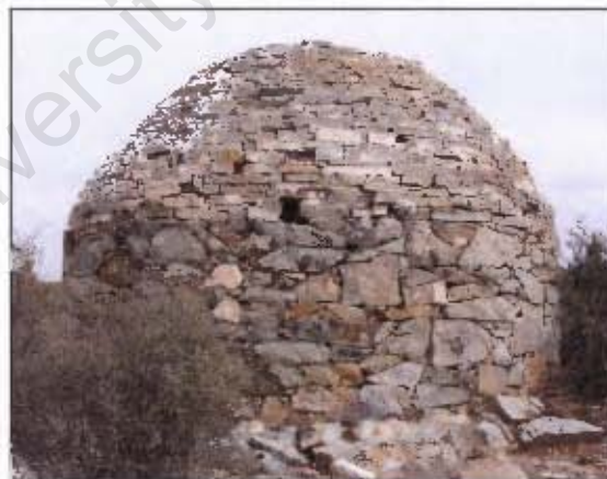
Figure 4.31 Koppiesfontein I. The wall of the kathok has a distinctive "crazy-paving" style.
