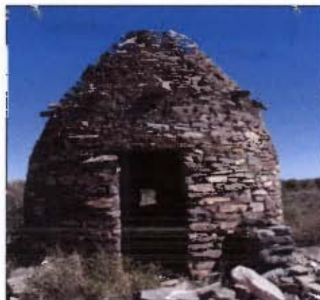
Figure 5.8. Omkeerkolk. The only oval base building located to date.
