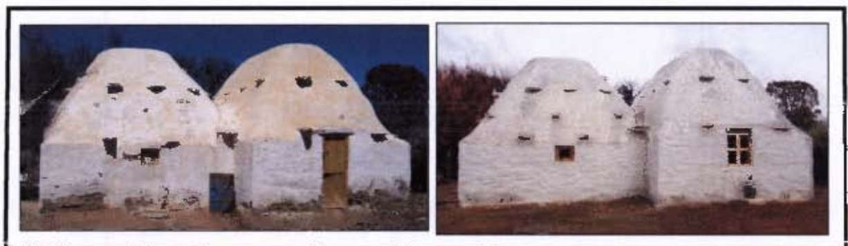
Figure 8.1 Droogeputs. Side view. The back door has been blocked and converted into a window ( right ). (Photograph on right: Judy Maguire.)
