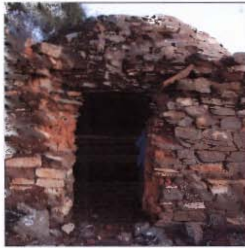
Figure 4.54 Aasvoelsvlei I. Brick-lined doorway which led into the later brick extension building
