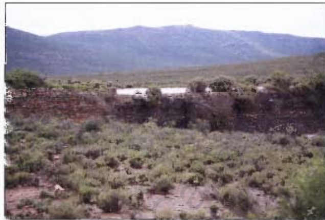
Figure 3.9 Large earth dam clad with stone built to block the river on Hondefontein.
