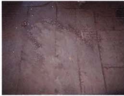
Figure 4.69 Vastrap. Floor laid with stone slabs.
