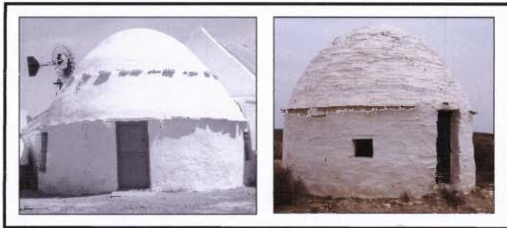
Figure 4.36 Krabfontein ( left ) and Modderfontein ( right ). Both have a stone ledge all around the building.
