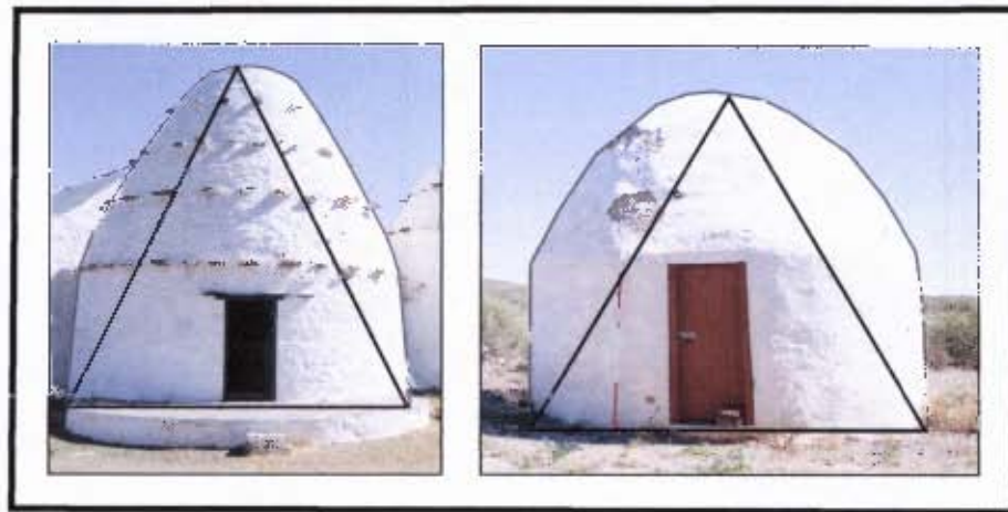
Figure 4.8 Illustrates the variability within the basic triangular shape of the round base corbelled buildings – Stuurmansfontein ( left ) and Dawidskolk ( right ).
