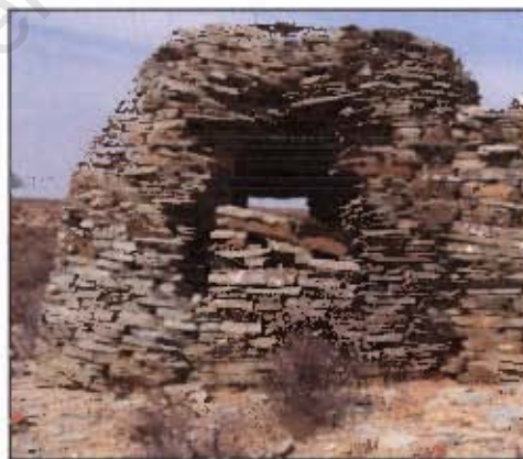
Figure 4.19 Aasvoelsvlei II. Broken stone window lintel.
