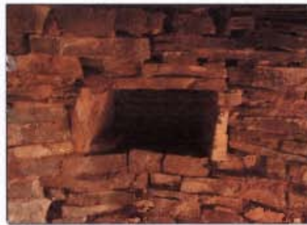
Figure 4.62 Aasvoelsvlei I. A simple wall niche (0.6m x 0.32m).
