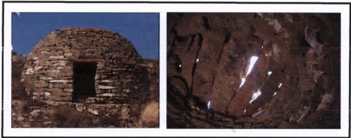
Figure 4.6 Mooskloof. The height to floor diameter ratio of 0.63 verges on an unstable semi-circle shape. The builder had to use five roof stones to close the roof hole.
