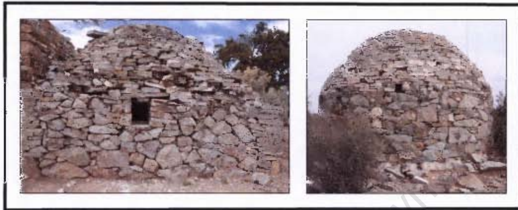
Figure 7.2 Koppiesfontein. Square base building ( left ) and round base building ( right ).
