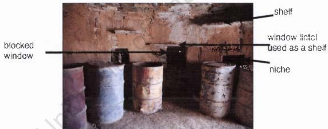
Figure 4.61 Brakvlei. Shelves, niches and a blocked window with a lintel which also served as a shelf.
