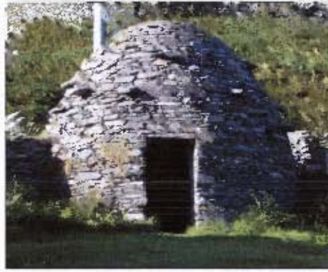
Figure 1.4 Corbelled building at Skellig Michael, Ireland, which would not be out of place in the Karoo.
