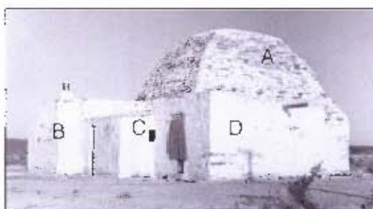
Figure 6.31 Arbeidersfontein. Walton's 1960 photograph of the corbelled building and three extensions, two of which have since been demolished (Walton, n.d.).
