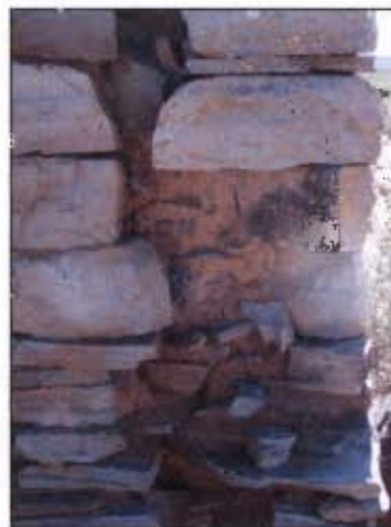
Figure 4.37 De Kolke. Mortar "hidden" in the wall.
