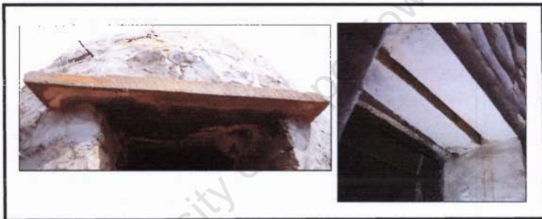
Figure 4.50 Onderplaas ( left ) and Arbeidersfontein ( right ). Onderplaas has a single large stone lintel, while Arbeidersfontein has two stone lintels.
