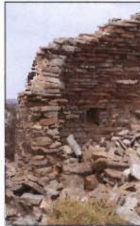
Figure 4.12 Boplaas. Section through the wall of a collapsed corbelled building shows the vertical double-skinned lower wall and the curved roof with its inward tilting layer of stones and outer revetment (Fig. 4.11).
