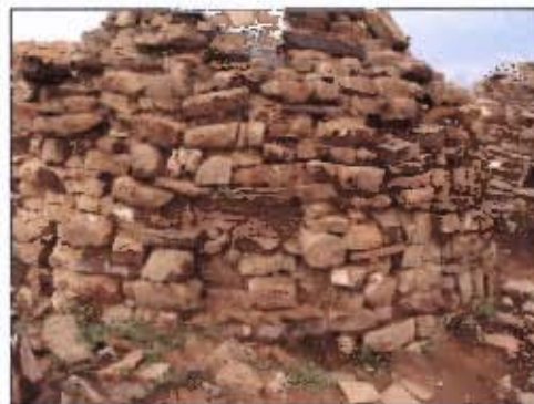
Figure 4.17 Krabfontein III. The use of uneven blocks of stone has led to collapse.
