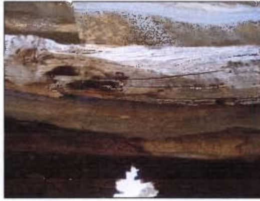
Figure 4.51 Stuurmansfontein III. Logs used for a lintel.
