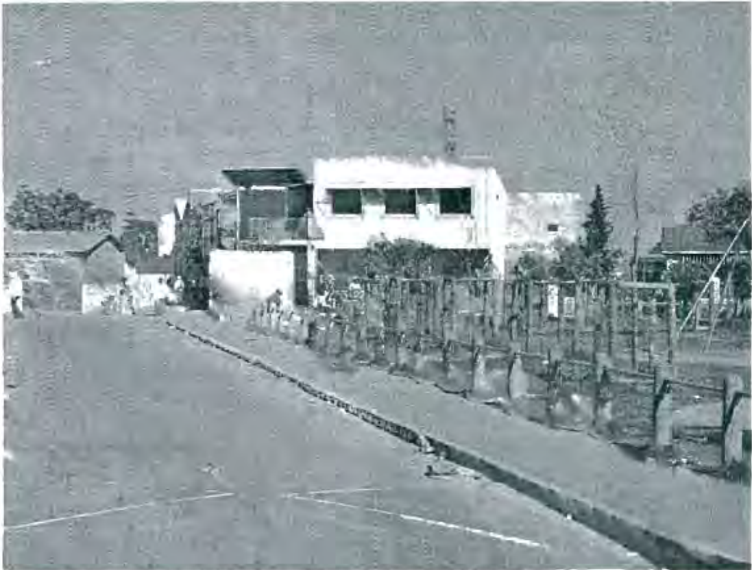
Photograph by author (1) Ulwazi youth centre Elevation North, Building phase 1. Site visit Langa 28/07/2004
