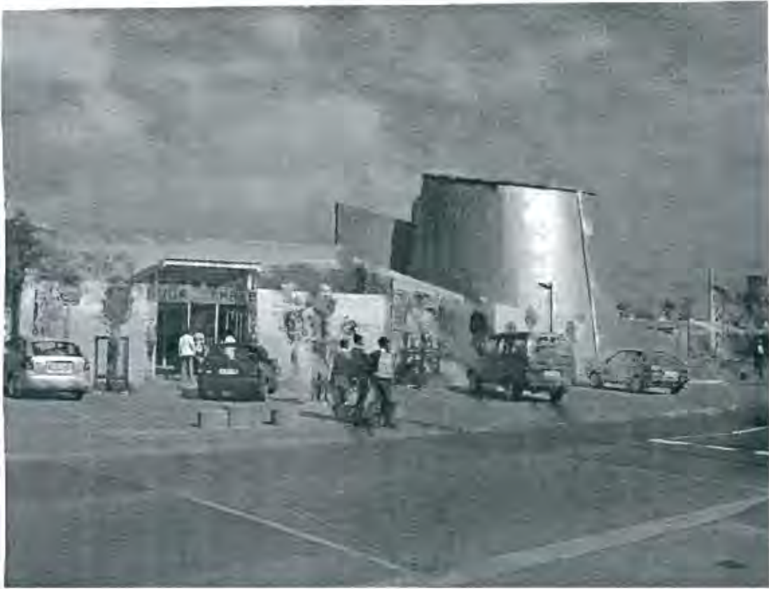
Photograph by author (5). Gugulethu Arts and Culture Centre, Elevation North, Site visit Langa 23/07/2004
