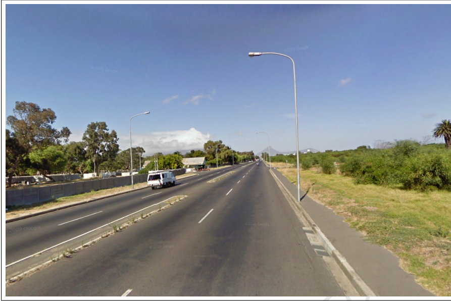
Figure 9.10: Undeveloped area along Voortrekker Road designated as cluster 5. To the left is a large cemetery, and to the right is an undeveloped strip of marshland. Source: Image sourced from Google Maps, accessed 15/04/2011
