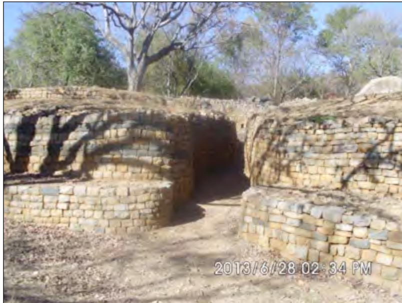
Figure 3.4: The Passage platform showing contrasting coloured blocks, on the left side, for aesthetic effect at the entrance to the platform.
