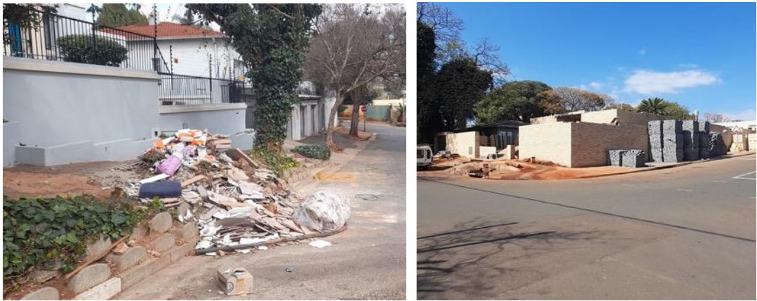
Figure A-25: Construction material outside residential properties
