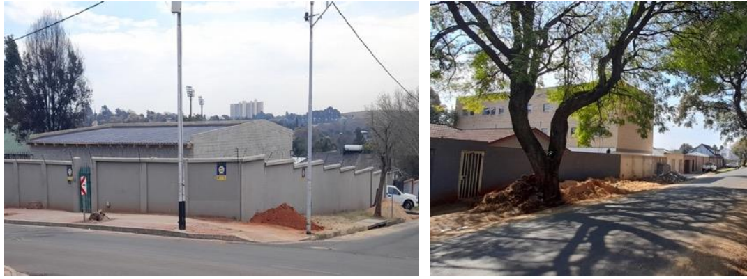
Figure A-15: Construction material outside private student housing properties
