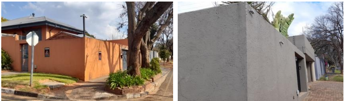
Figure A-44: Private security measures at properties
