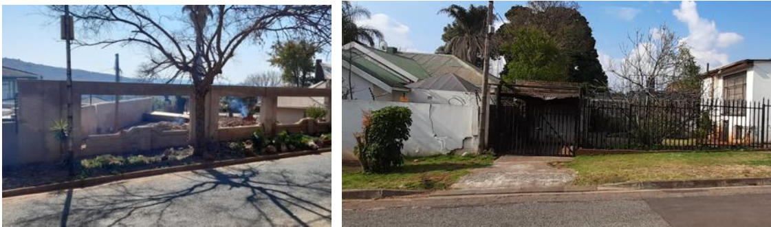
Figure A-28: Dilapidated residential property
