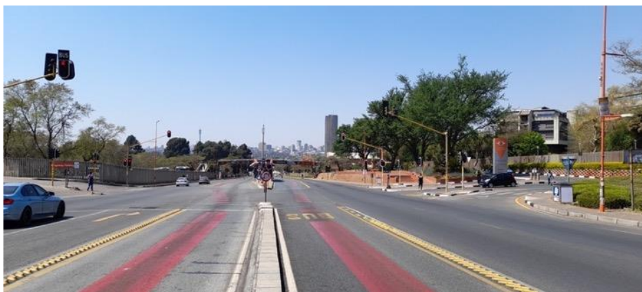
Figure A-5: UJ APK Campus off-campus student parking facility (left) with a pedestrian bridge (background) leading to the campus (right)
