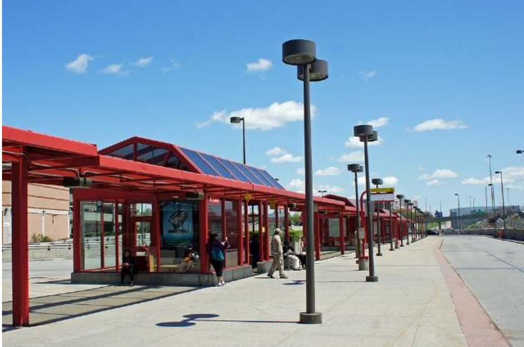
Figure 50. Typical transitway station in Ottawa (St. Laurent station). Source: http://www.wikiwand.com/en/Ottawa_Rapid_Transit .
