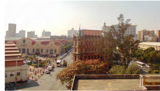
Fig. 2.2: The Old Durban Railway Station Building and the Workshop
