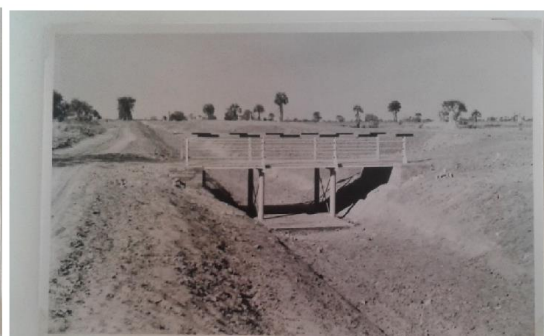
A “so called” canal bridge crossing for men and cattle. Such a bridge is constructed more or less every 4 miles.
