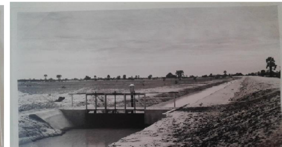
A “so called” canal bridge crossing for men and cattle. Such a bridge is constructed more or less every 4 miles.
