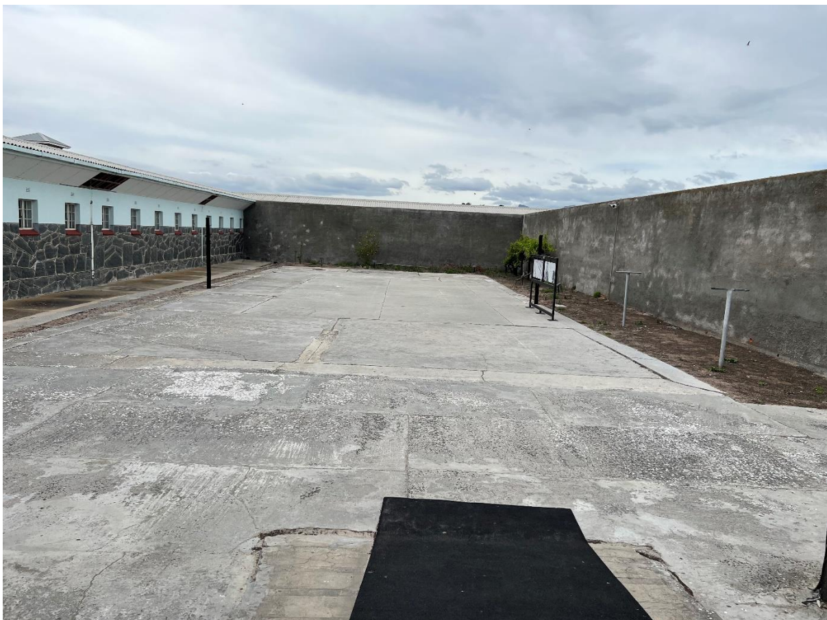
Figure 30: Section B courtyard with single cells in the background
