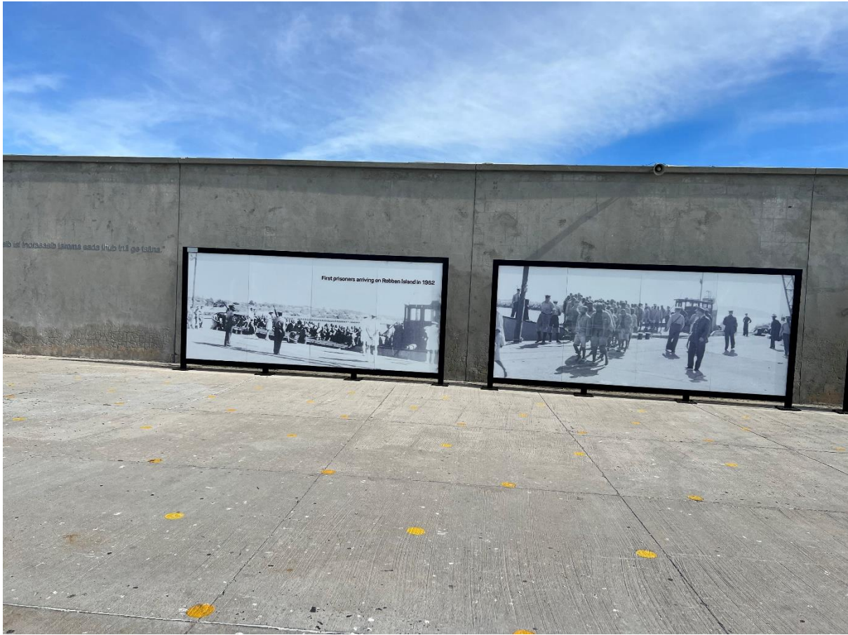
Figure 16: Murray's Bay harbour. Part of the wall was constructed during WWII era using remnants from leper buildings.
