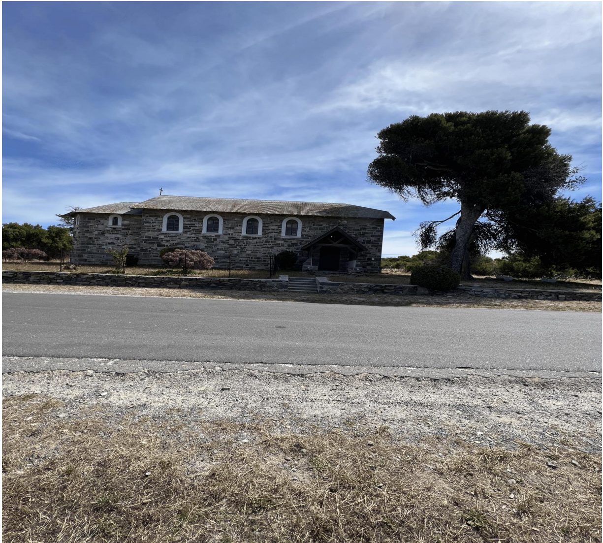
Figure 4: Side views of the Good Sheppard Church (source: Author 2021)
