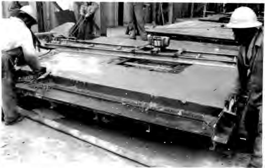
"MUST" SYSTEM - (d) Vibrating screed finishing
