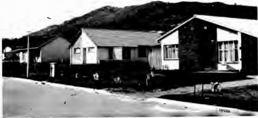
Some of the first houses, built departmentally.
