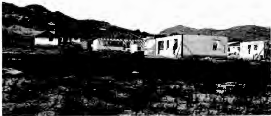
New houses under construction, 1972 ; part of a 179-house contract.
