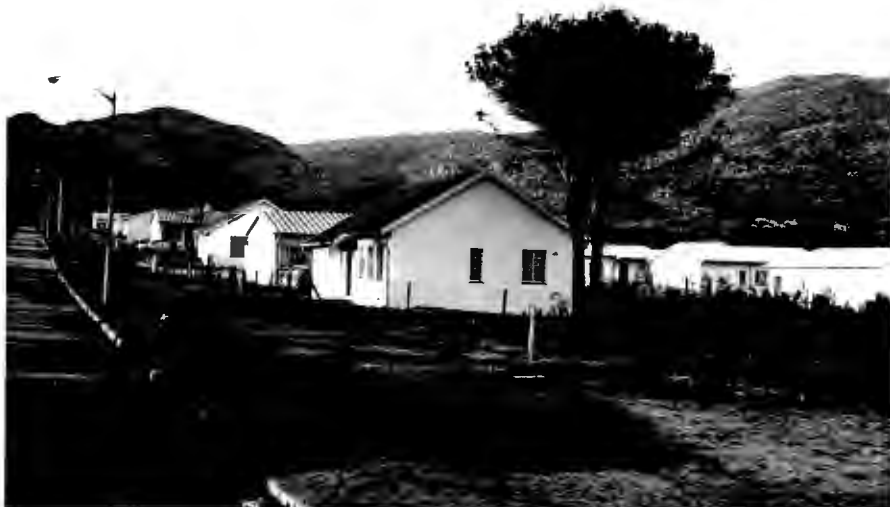
A street of no-fines houses after completion of the 82-house contract.
