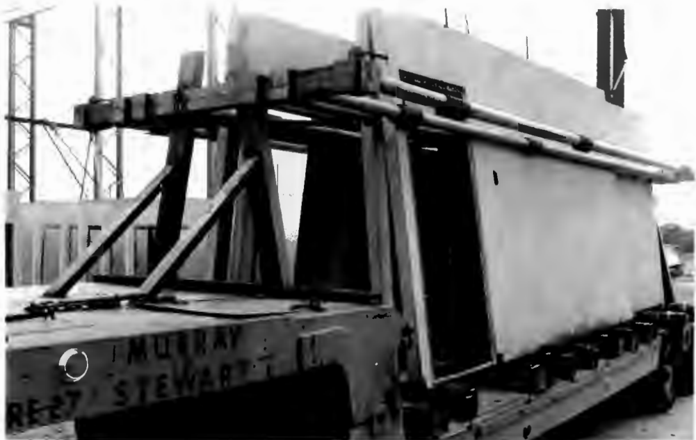
"MUST" System - (f) Wall panels on the "toastrack" trailer.
