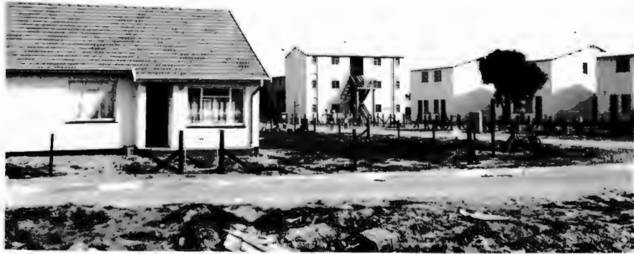
GRASSY PARK EXTENSION 10 - From left to right, single house (selling scheme), 3-storey block of flats (letting), double-storey maisonettes (letting). All contract built.
