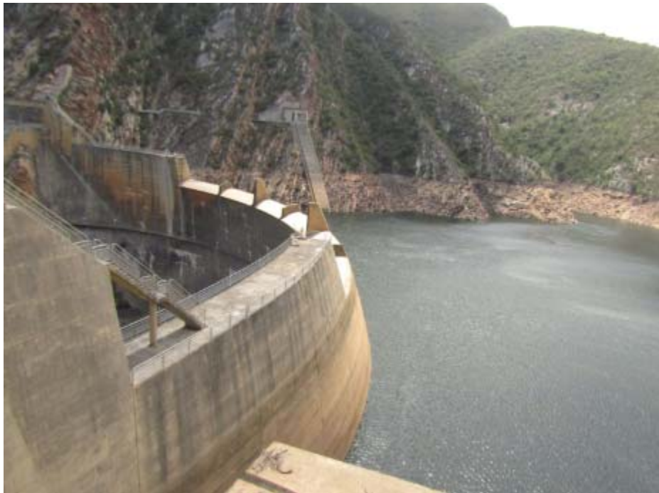
Figure 2.1. Kouga Concrete Arch Dam
