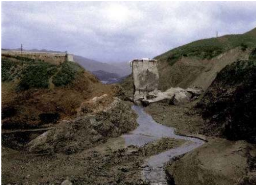
Figure 1.1. St Francis Lake Dam after failure (Rogers, 2007)
