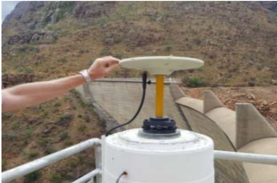
Figure 5.4. GPS receiver on the dam crest
