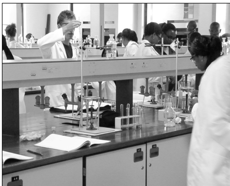
Figure 8.1 Photograph showing the service duct running along the length of the laboratory bench.
