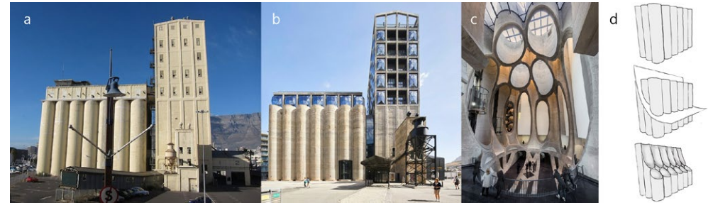
Figure 83: A sequence of images illustrating how the original grain silos at the V&A Waterfront (a) were structurally modified (d) to become the museum and hotel that they are today (b-c).
