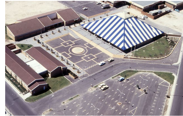
Figure 66: aerial view photograph taken by G. Parker of the first pyramidal structure built in Mitchells Plain, Cape Town.
