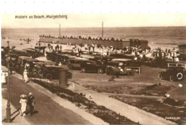
Figure 35: the formal garden built between the first pavilion and buildings beyond (figure 33) was converted into a parking lot when the motor car gained popularity in the 1920's and established a need for parking which was not originally anticipated (Gasson, 2019, p.52).
