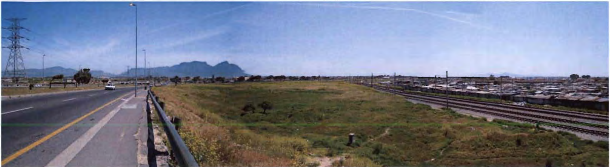
4.20 View down Lansdowne Road bridge towards West, with railway line on the right
