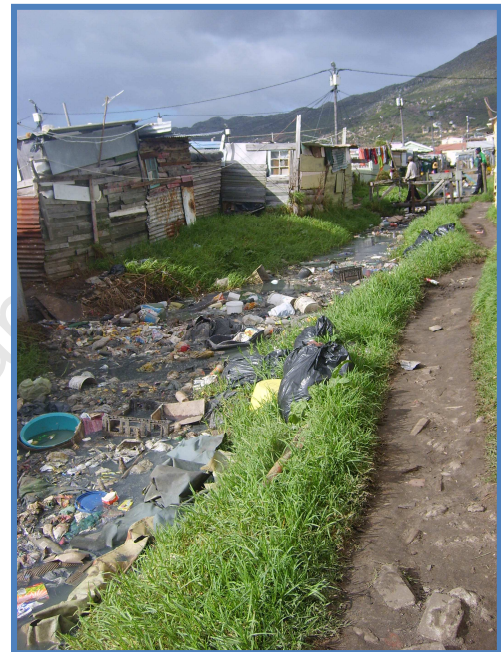
One of the clogged Drainage Channels – Wetlands
