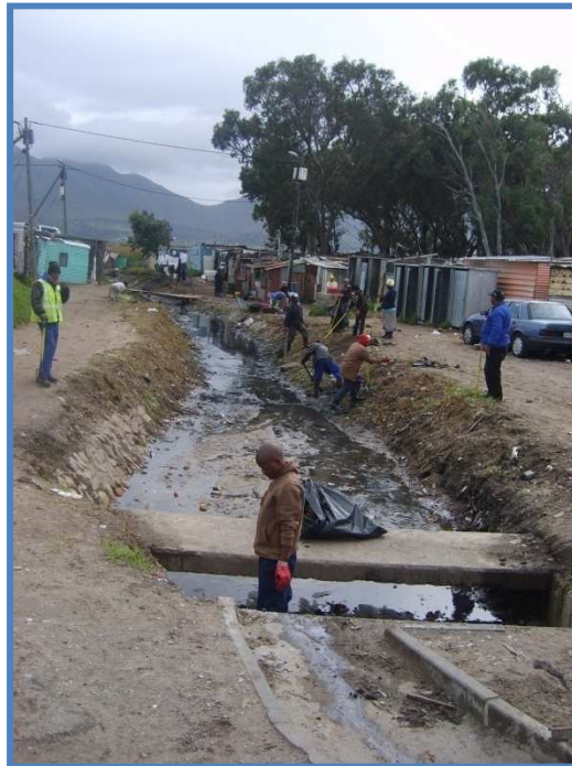
Figure 6.6 City of Cape Town Contractors clearing Drainage Channels in Masiphumelele
