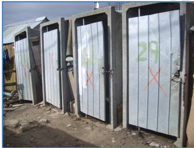
Figure 5.19 Toilet Facilities in Wetlands area
