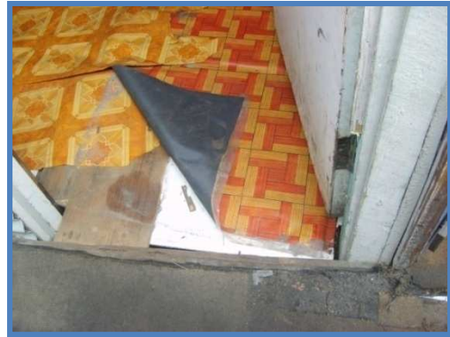
Mitigation Measure: Plastic Linoleum Covering the Floor of a Dwelling - Wetlands
