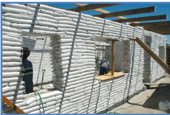
Figure 6.4 Example of a Sandbag house being constructed in Masiphumelele
