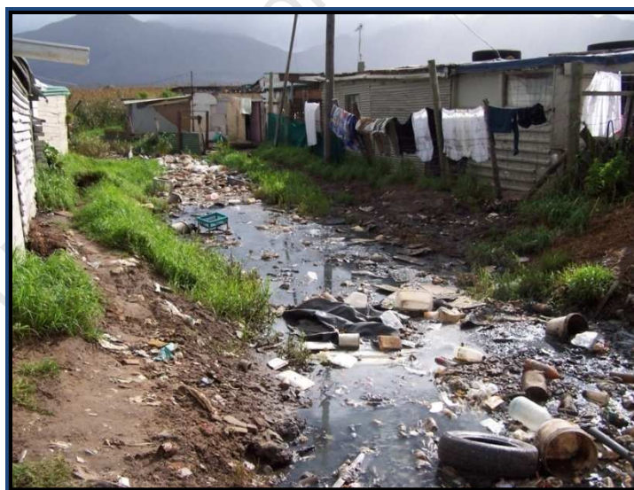
Figure 5.23 Homes in Masiphumelele built close to drainage channel
