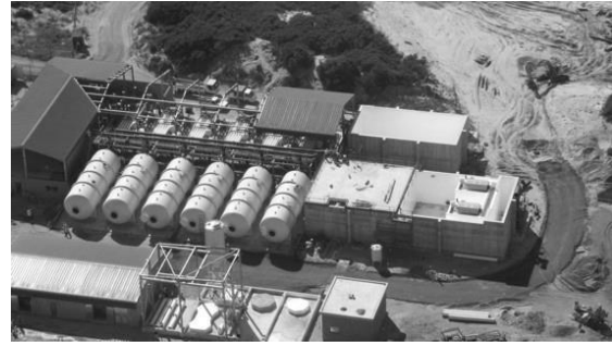
fig. 72 Mossel Bay Desalination Plant
