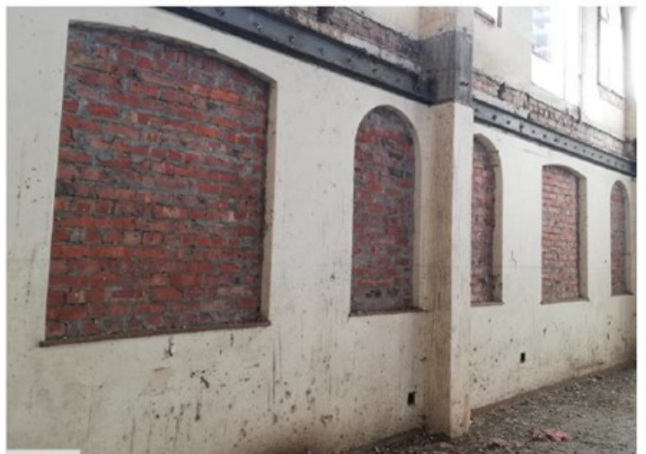
Figure 33-38: Gutted interior of existing building (Rigsby, 2019)
