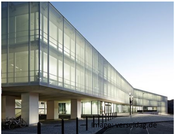
Figure 65 & 66: The Fritz-Lipmann-Institute's (by HKS Architekten) PTFE glass mesh fabric façade. This white mesh is used as interior space-making element, creating a white canvas interior. (Concrete Structures NZ LTD, 2022)
