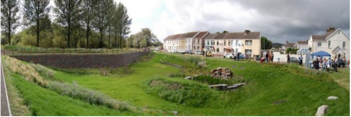
Figure 2-8: Vegetated detention pond (Welsh Water, 2017)
