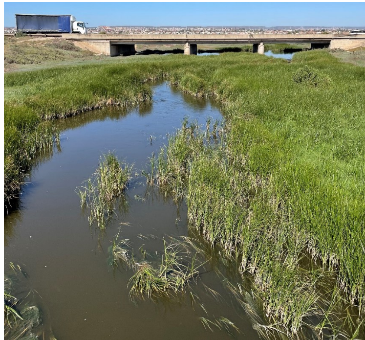
Figure 6-17: Channel with dense vegetation at Site 1 (Chatty Outflow) (20 th October 2021)
