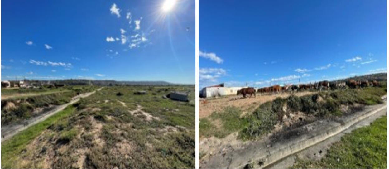
Figure 8-7: Semi-circular concrete channel
