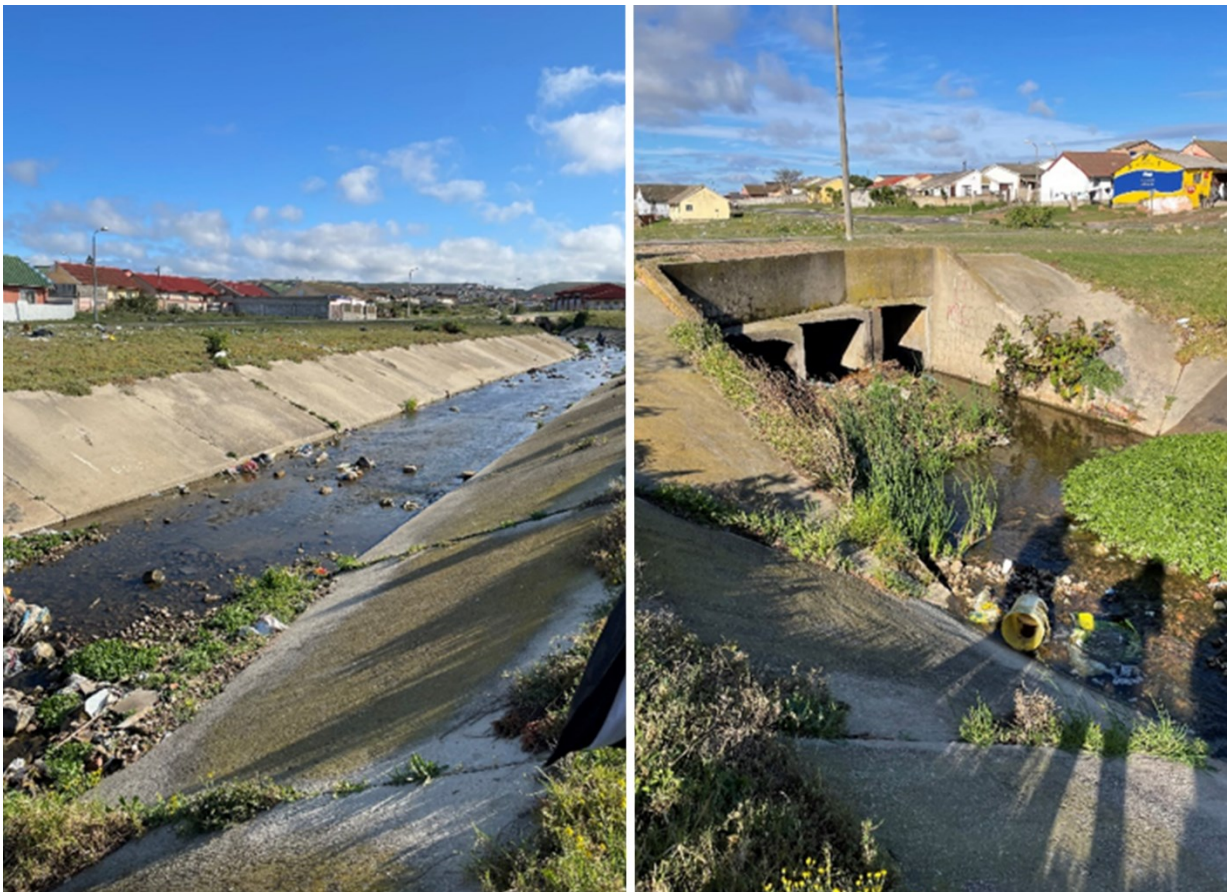
Figure 5-11: Trapezoidal channel at Site 14 (Bethelsdorp)
