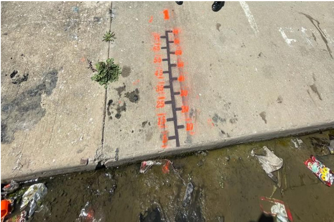
Figure 5-12: Stencil placement on the slope of the trapezoidal channel
