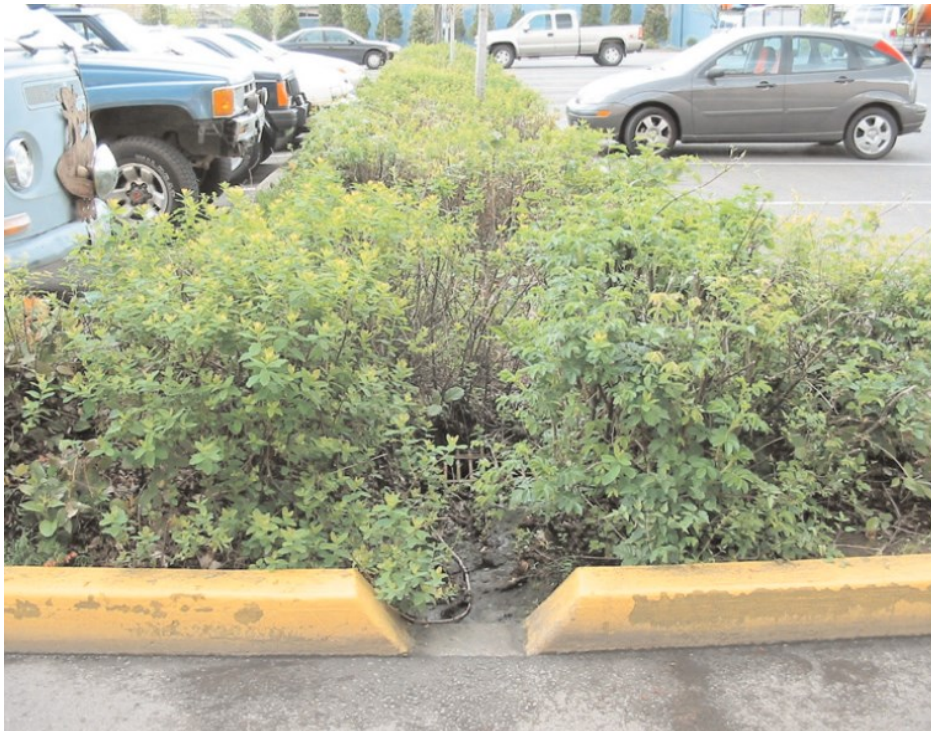
Figure 2-7: Example of bioretention application in a parking area(Ballard et al. , 2007)
