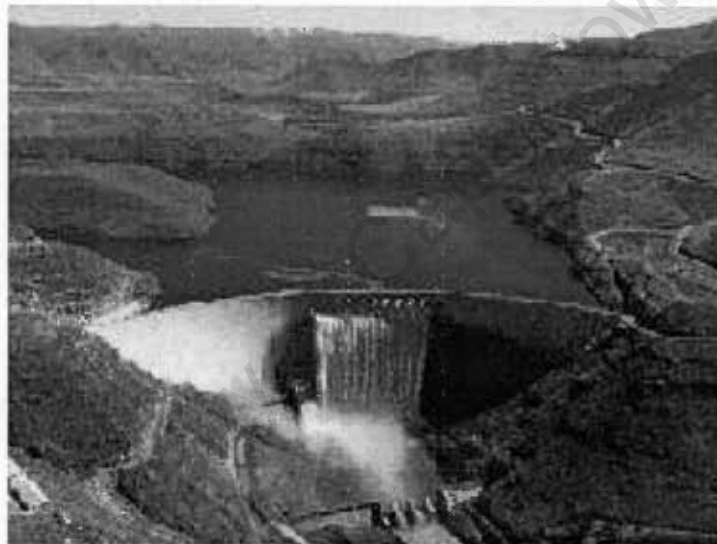
Figure 2: Katse Dam, 1 st of 5 Dams in the Lesotho Highlands Project
