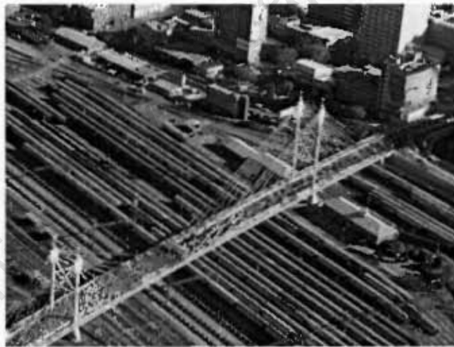
Figure 4: The Nelson Mandela Bridge
