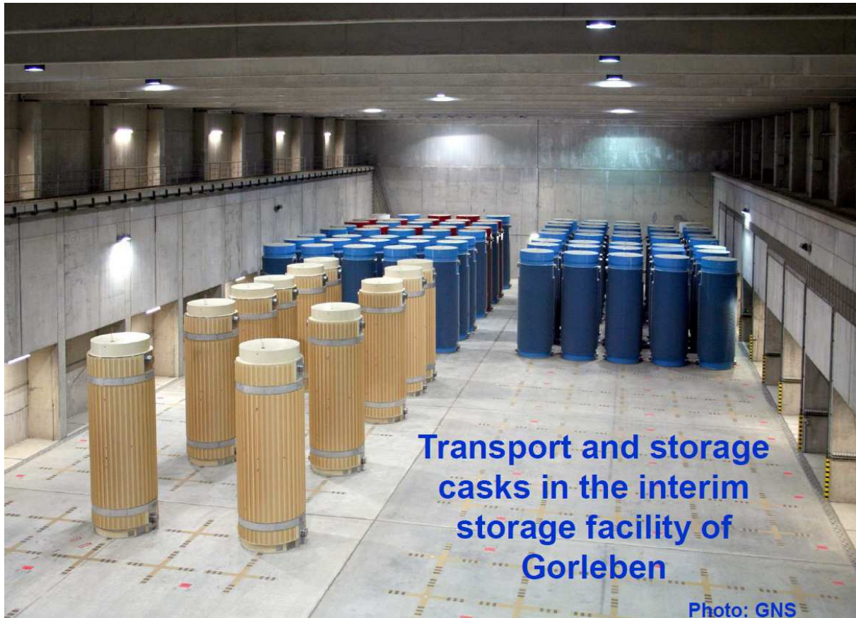
Figure 22: Transport and storage casks in the concrete interim storage facility of Gorleben, Germany (Sanono, 2013)
