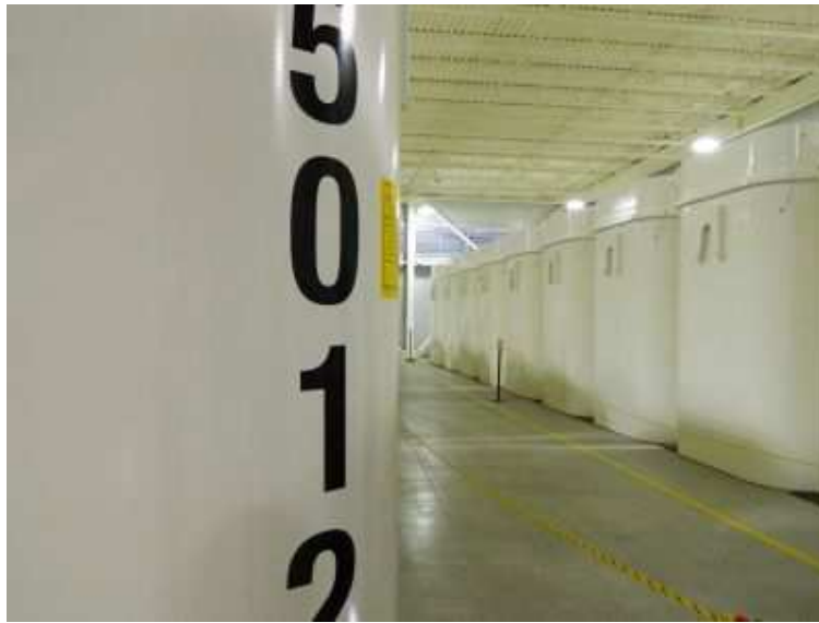
Figure 20: Concrete pad with cladded-type enclosure structure as ISFSI facility (Reddit, 2010)
