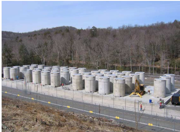
Figure 18: Dual purpose canister system on concrete pad, ISFSI at Connecticut, Yankee (D. Vinson, 2011)
