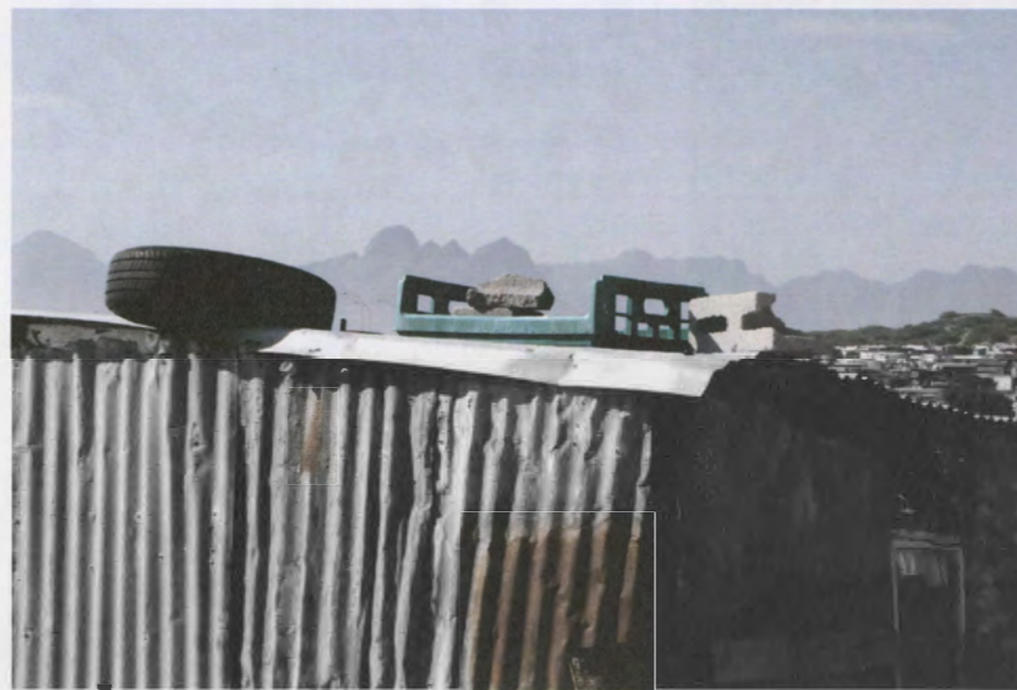
Various useless objects provide weight to the roof
