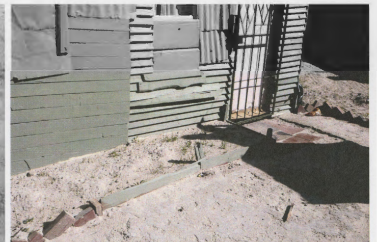
embankment protected by brick box
