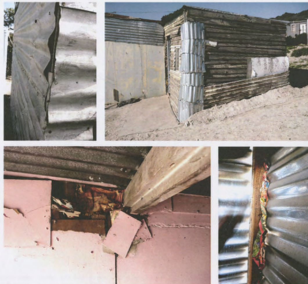
closing the gaps to stop sand from getting into the house
