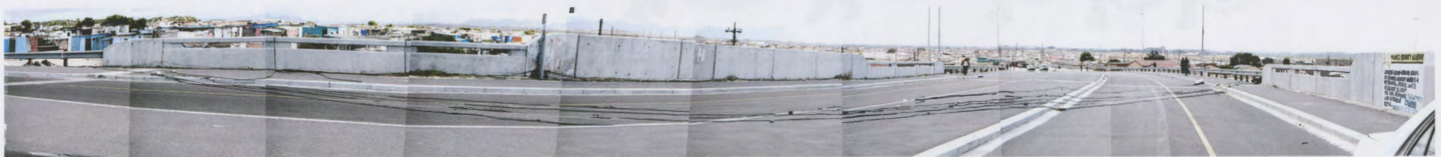
Electric cables cross Walter Sisulu Bridge
