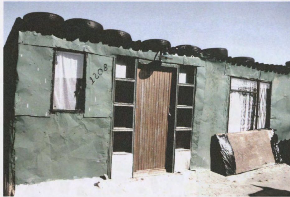
Tyres protect roof
