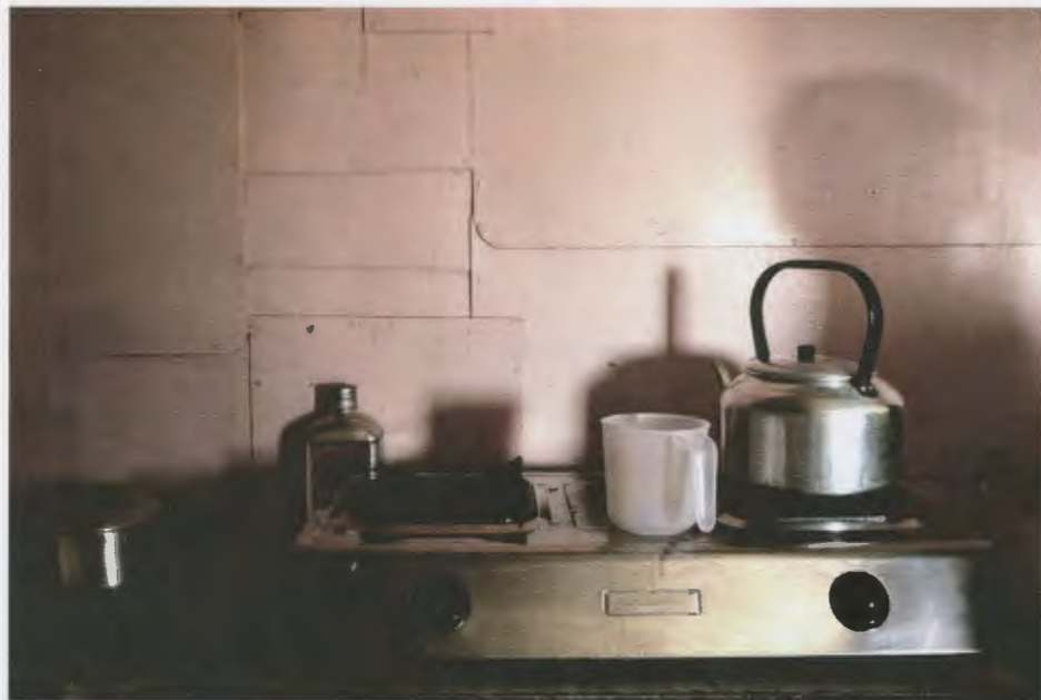
Gas stove safer than kerosene one. stove very close to inflammable timber boards
