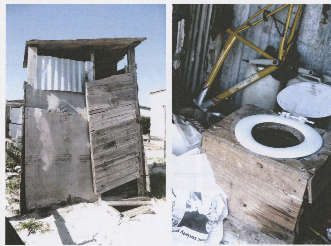
Inside and outside of a toilet
