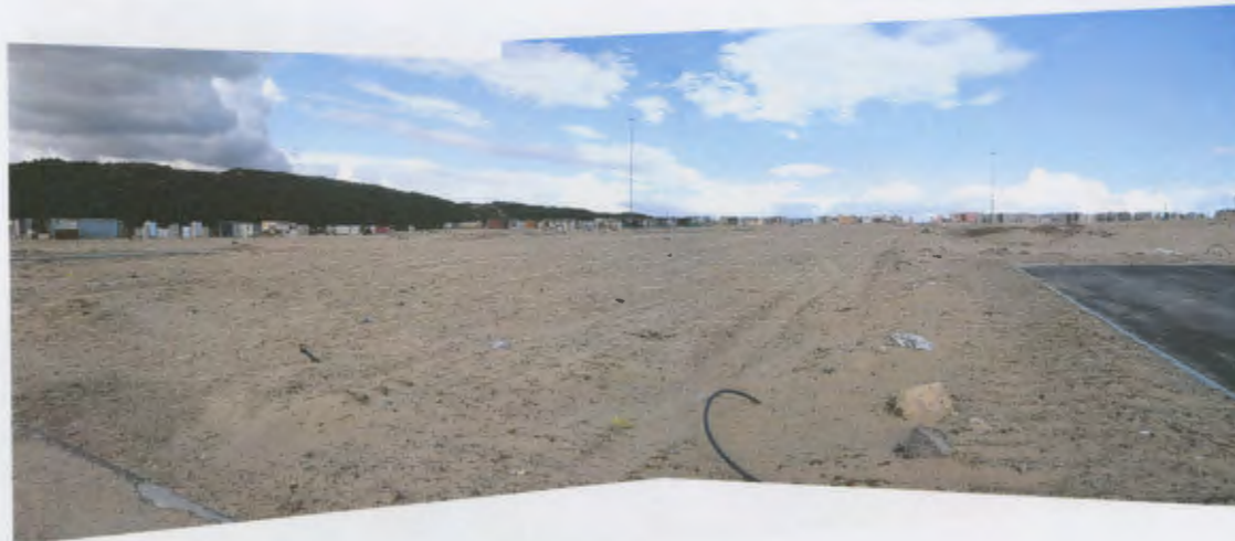
Photo of Zwelitsha in the process of being constructed
