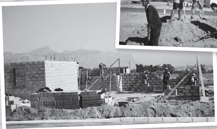
BELOW The first houses being erected.
