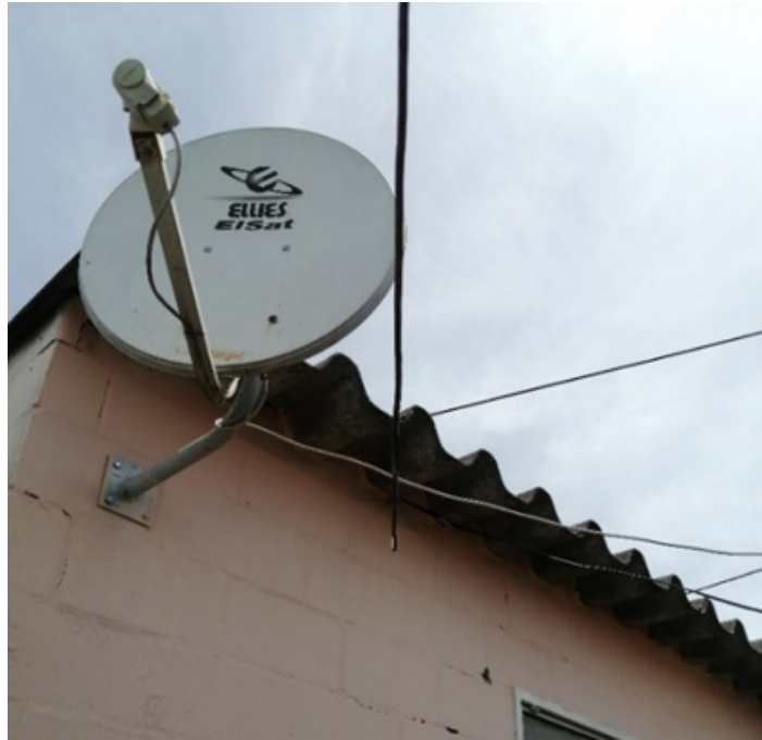
Image 24: Illegal electric connections. Source: Author (2022)
