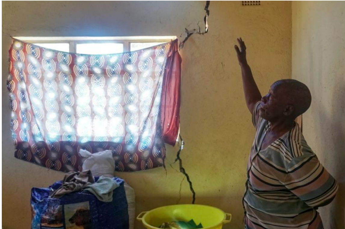
Figure 4 House built by Anjin in Arda Transau
